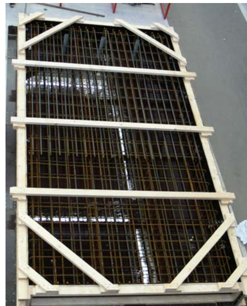
Formwork and reinforcement for slab experiments
